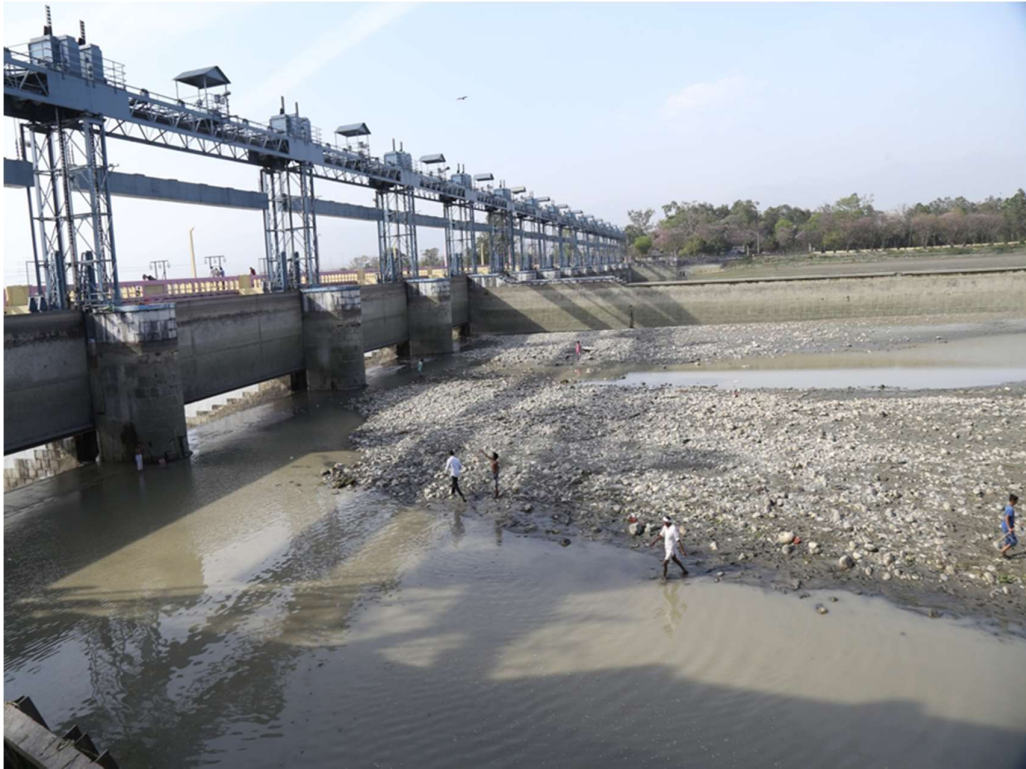
De-silting work under sluice gate side before start of closure
