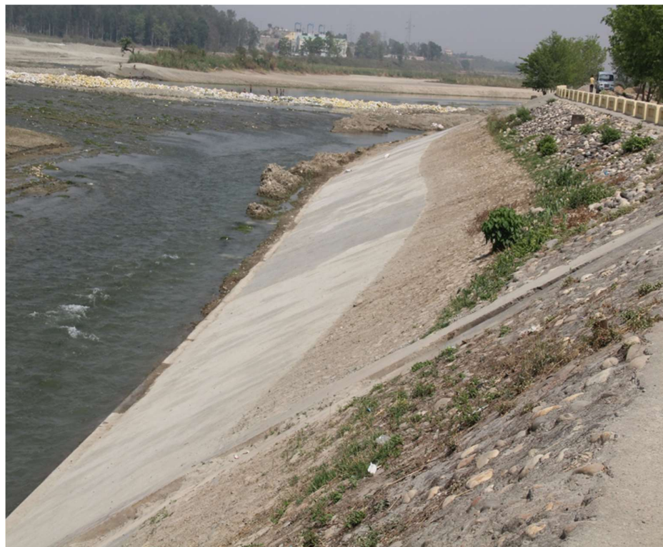
Left Bank of Asan reservoir after completion of closure work
