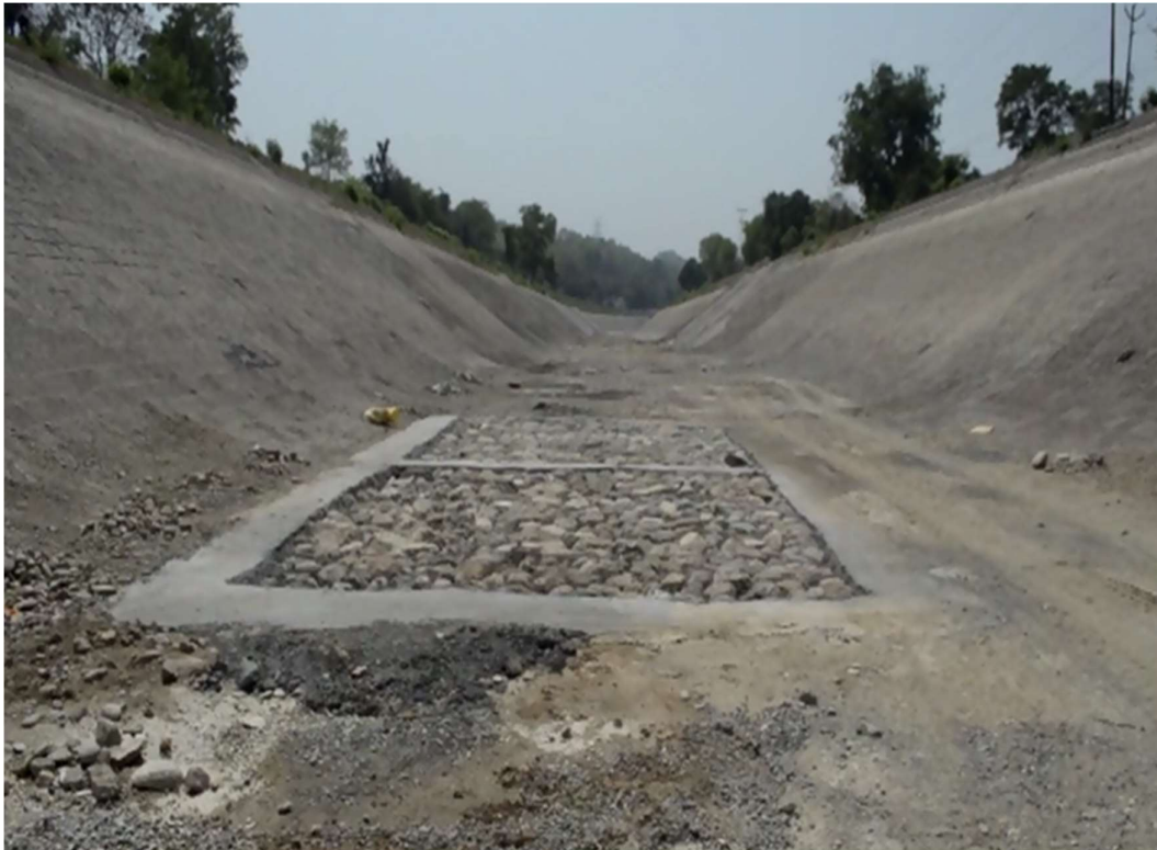
Channel bed Near Bridge No 2 after repair
