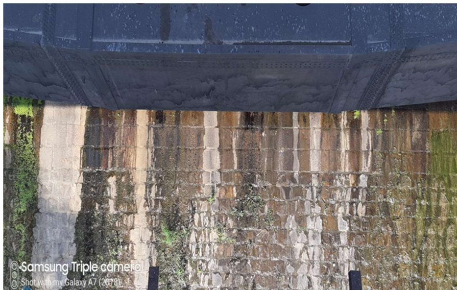
Barrage Gate after bottom rubber seal replacement
