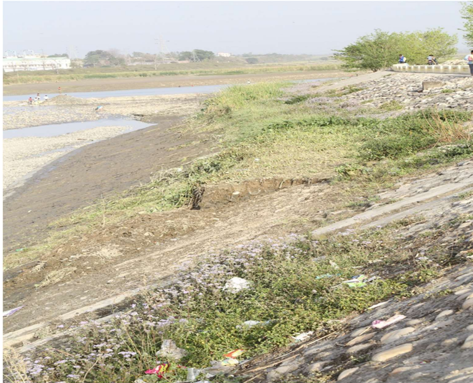
Left Bank of Asan reservoir before start of closure work
