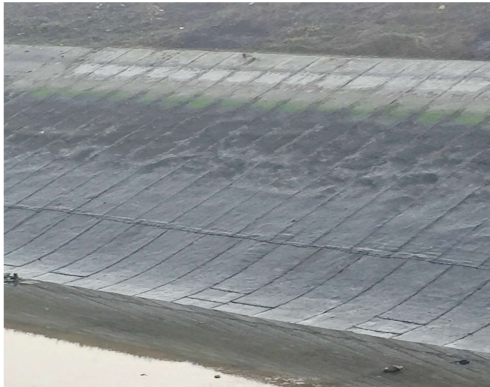
Laying of Concrete canvas over the bank of Power Channel
