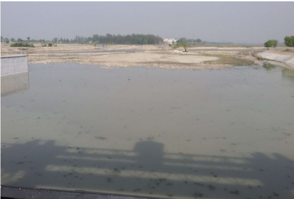
De-silting work under sluice gate side after finishing closure work
