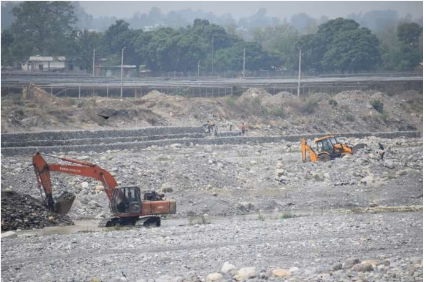
Status of protection works at downstream left bank after repair works
