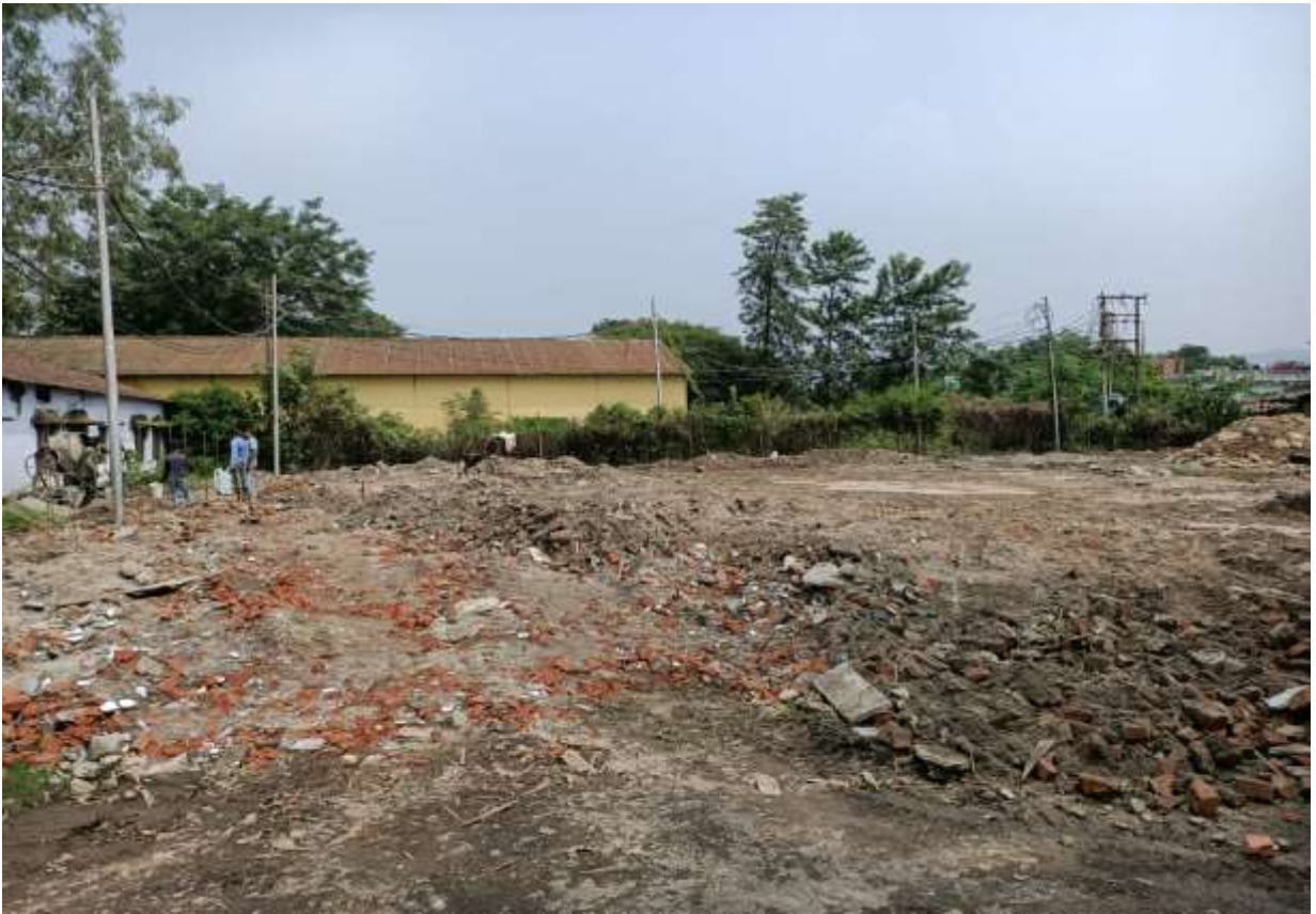
Construction site office building at Dakpathar
