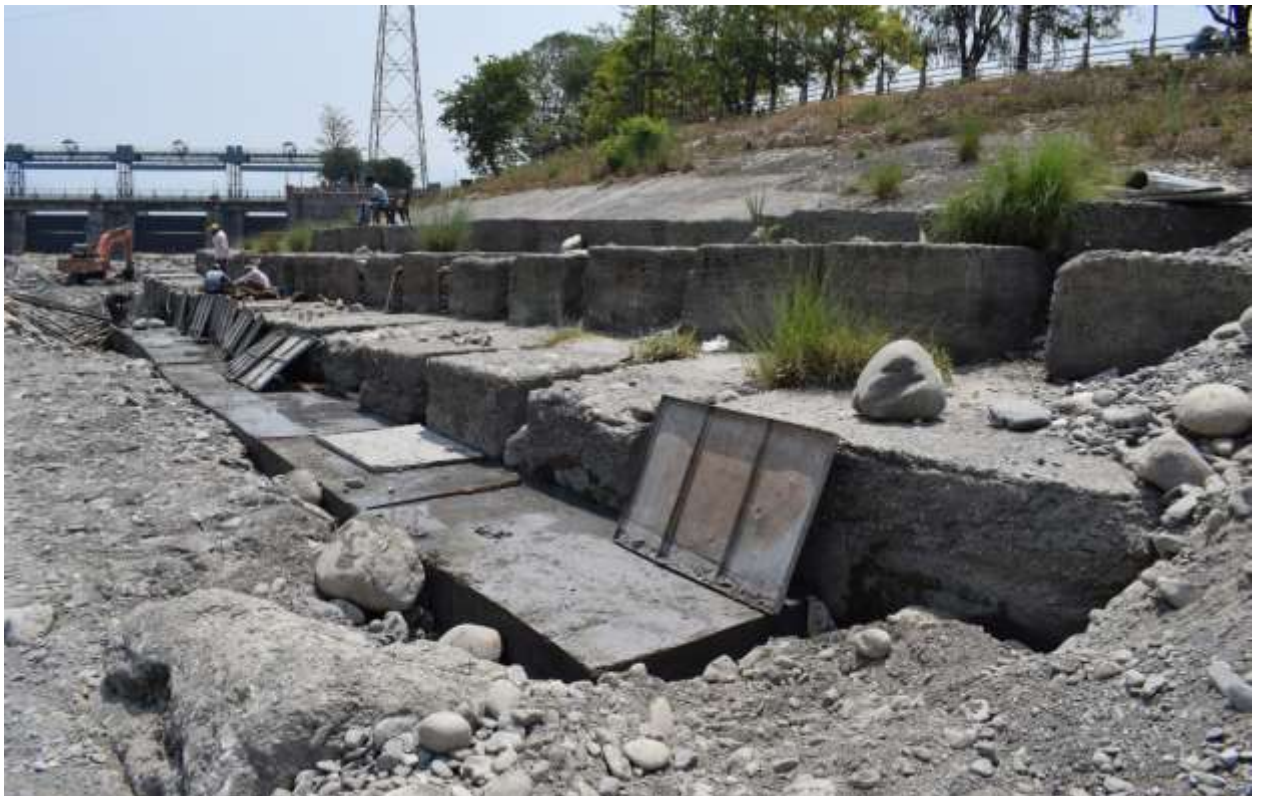
Status of protection works at downstream left bank after repair works
