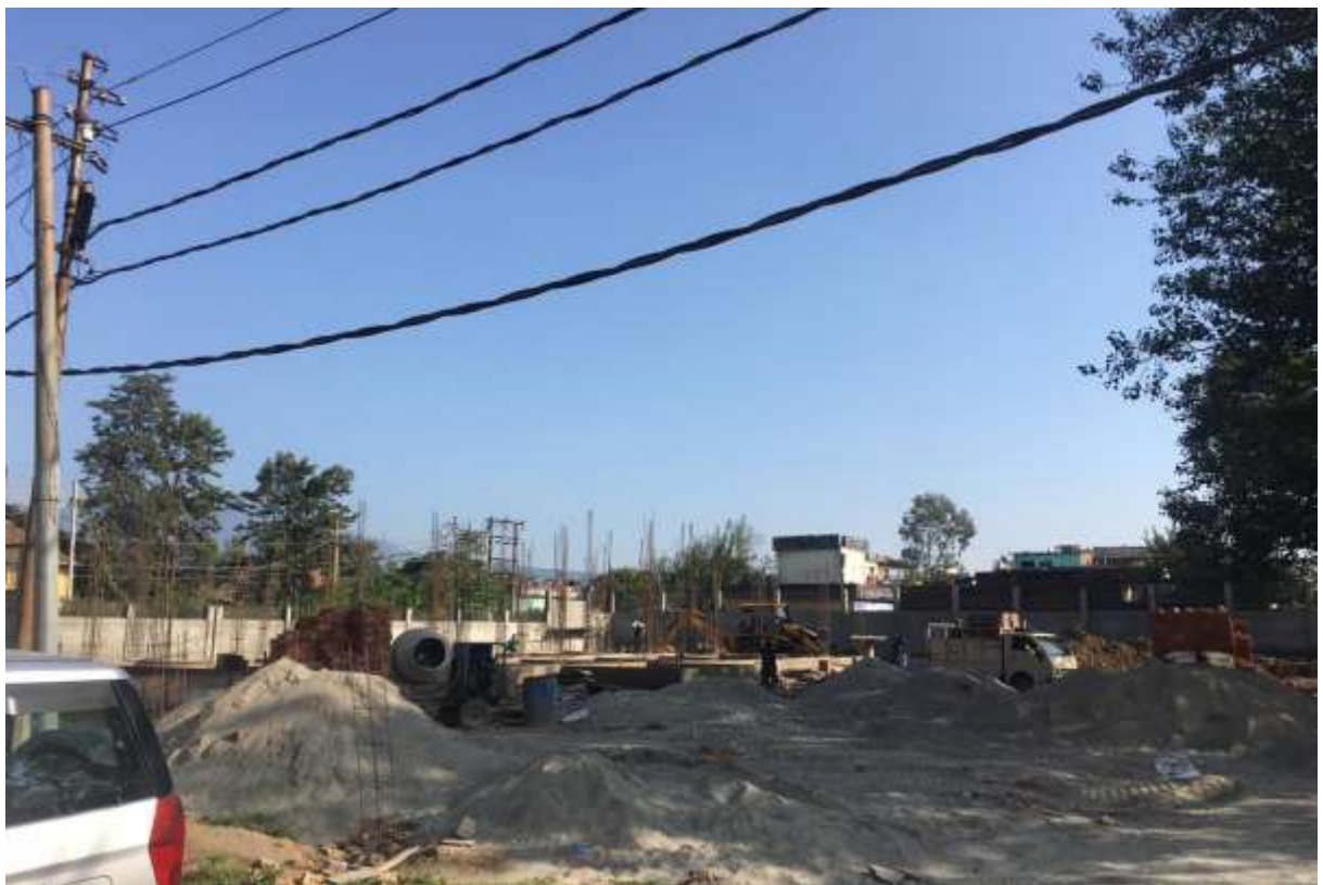
Under construction office building at Dakpathar
