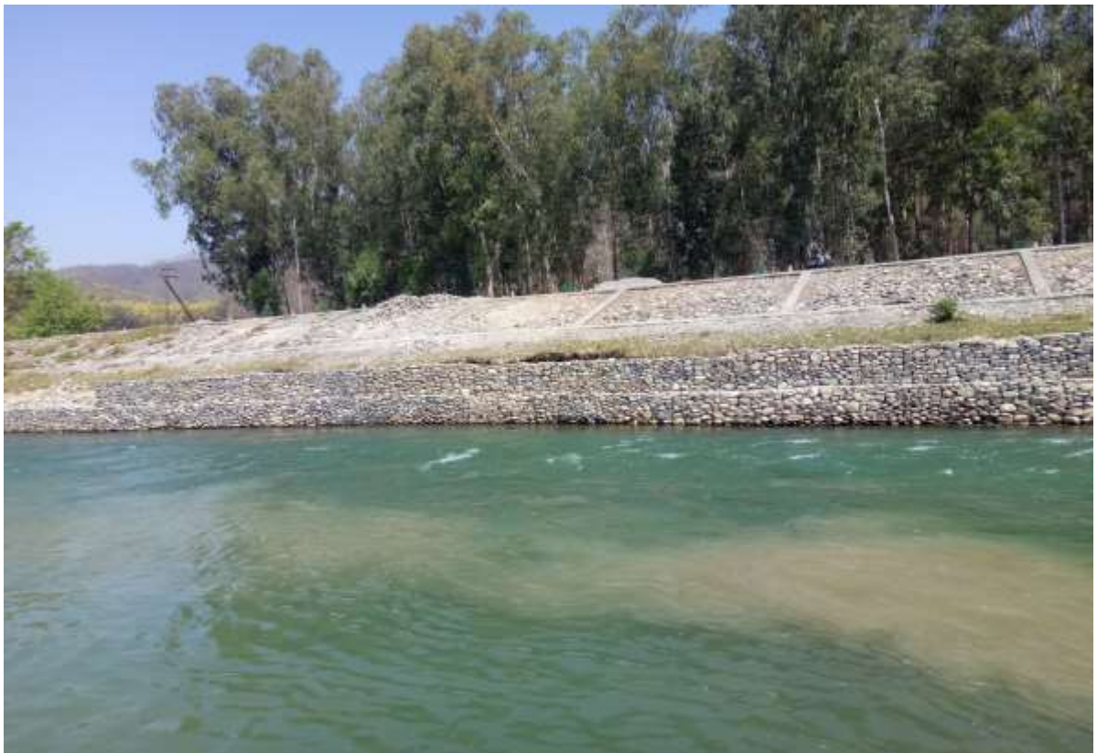
Status of upstream right bank after repair works
