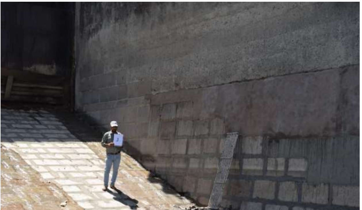
Status of downstream glacis & piers after repair works
