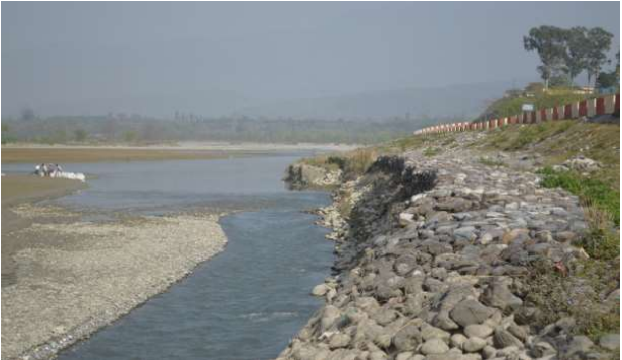
Status of upstream left bank before repair works
