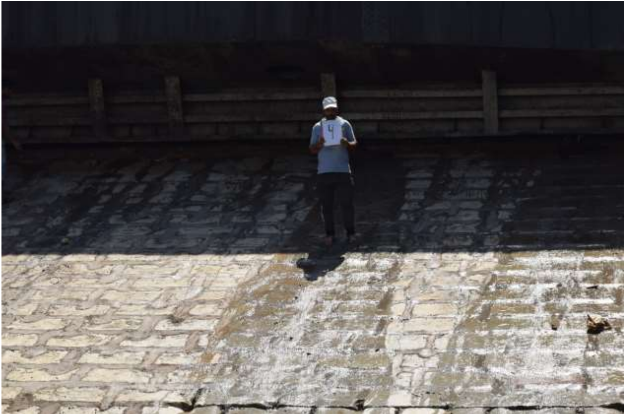
Status of downstream glacis after repair works
