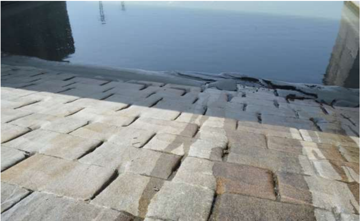
Status of downstream glacis before repair works
