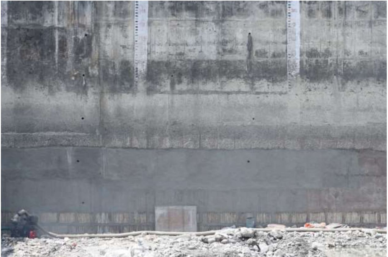
Status of abutment at gate no 1 after repair works at downstream
