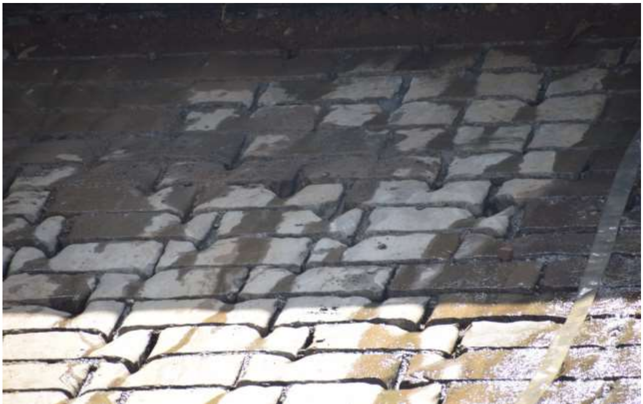
Status of downstream glacis before repair works
