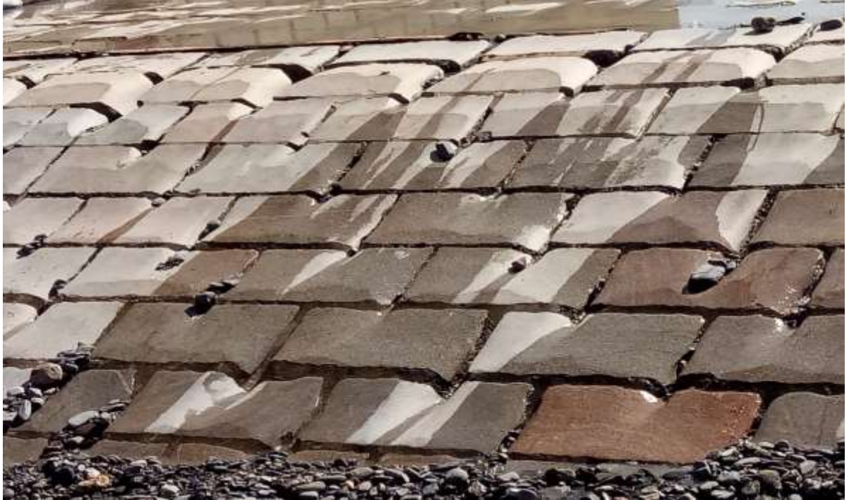
Status of upstream glacis before repair works
