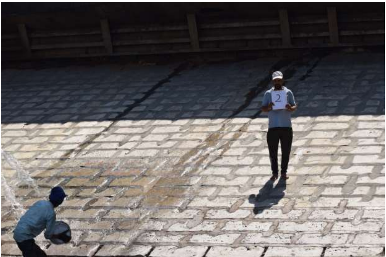
Status of downstream glacis after repair works
