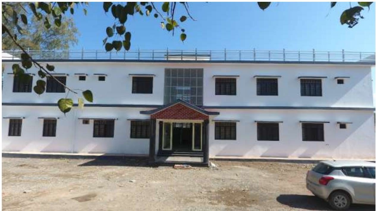
Front View of office building
