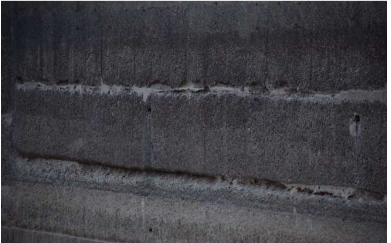
Status of abutment at gate no 1 before repair works
