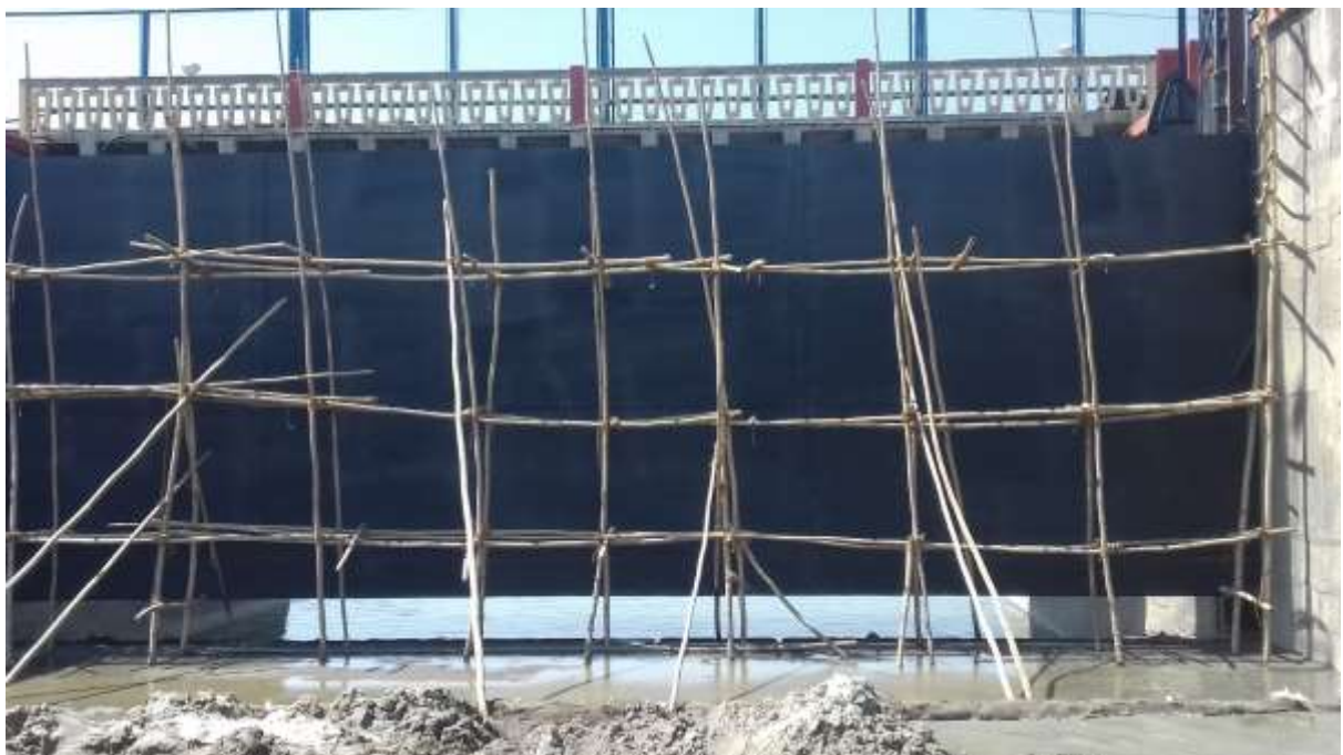
Barrage gates after epoxy painting
