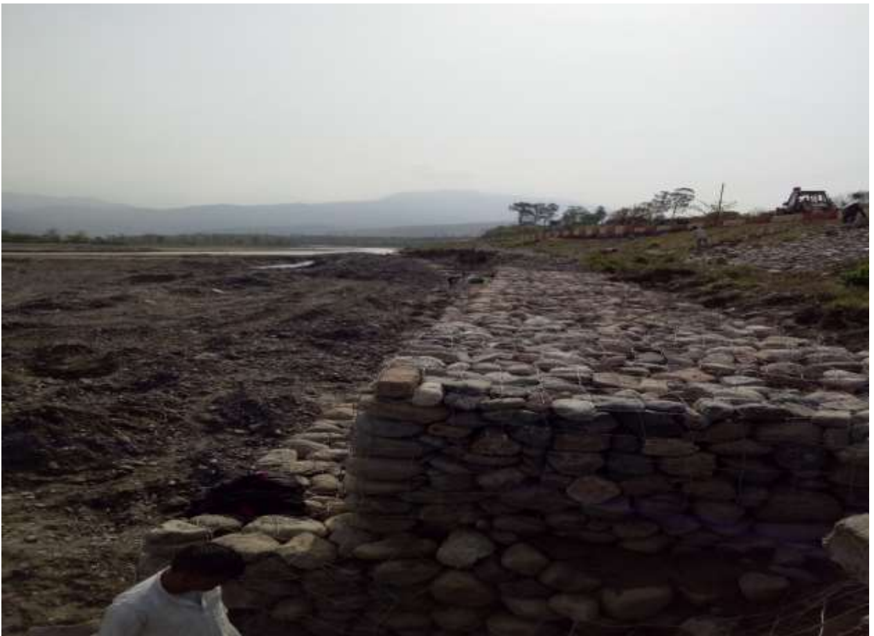
Status of upstream left bank after repair works
