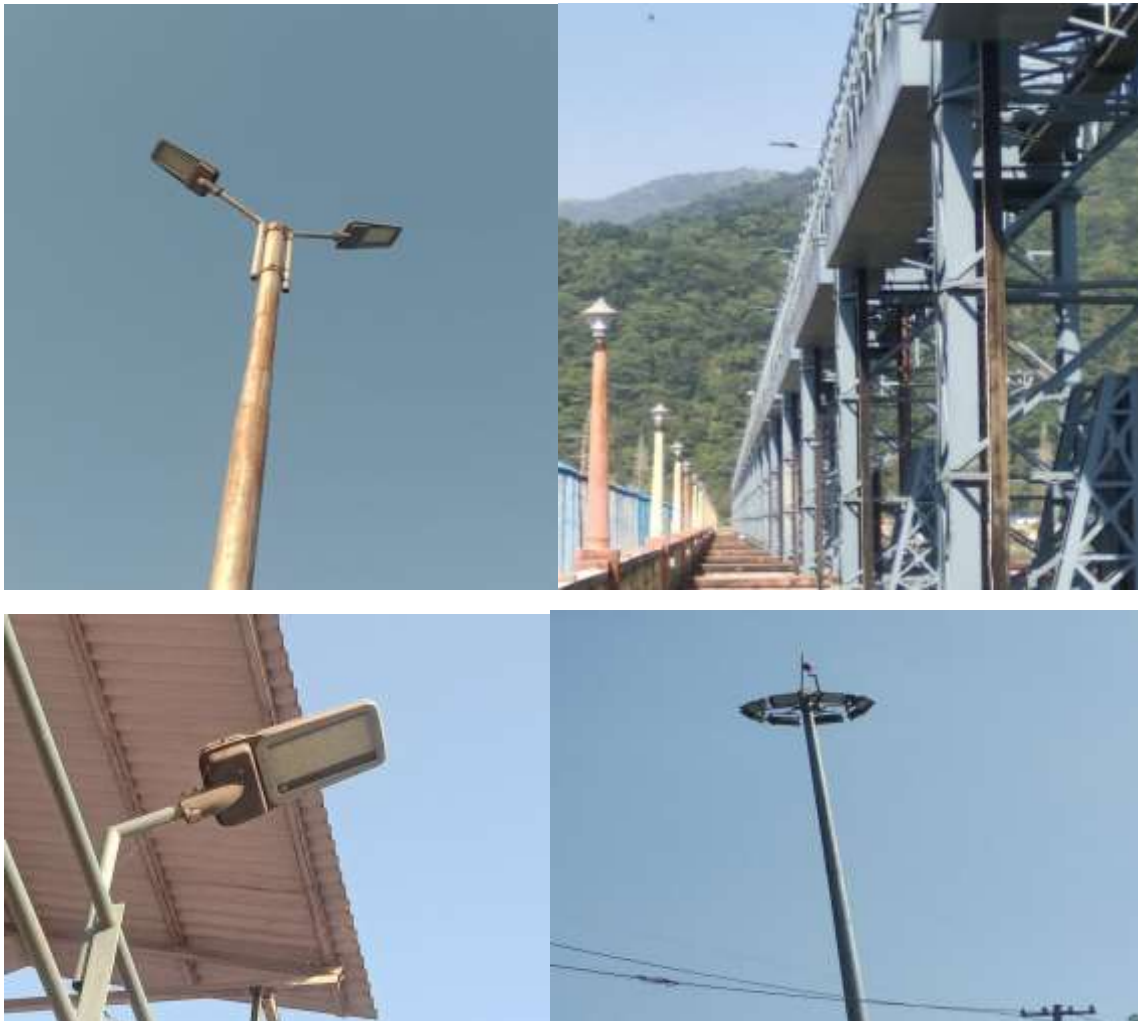
LED's (luminaries) after installation
