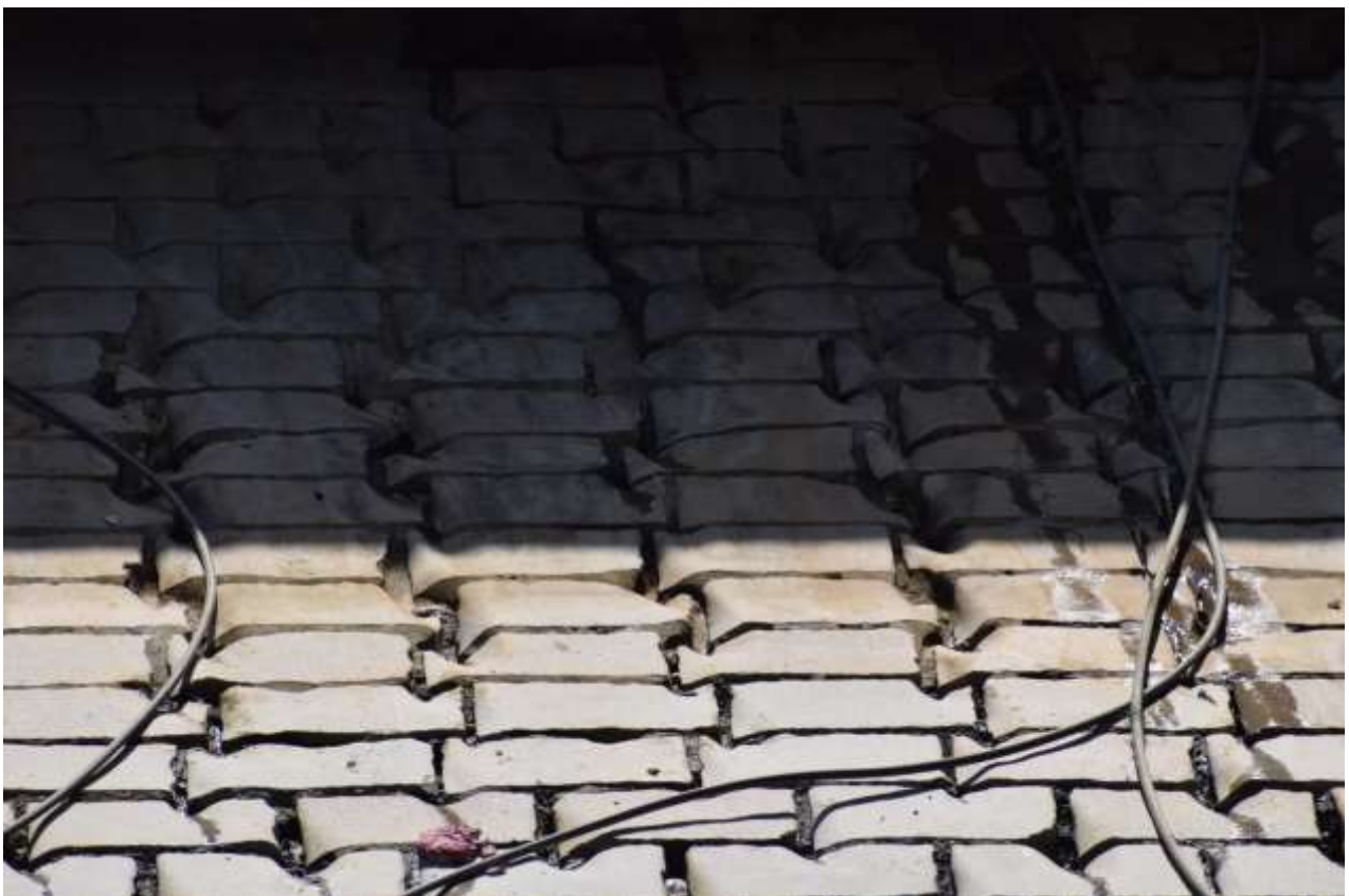
Status of downstream glacis before repair works
