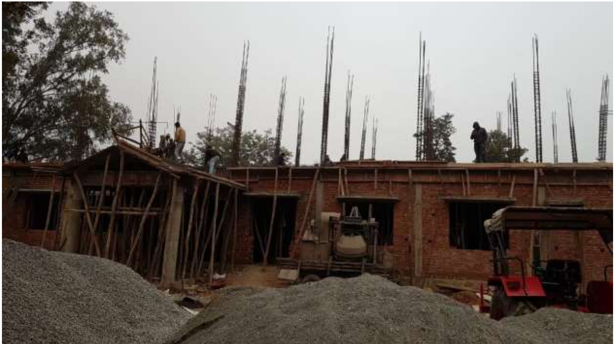
Under construction office building at Dakpathar
