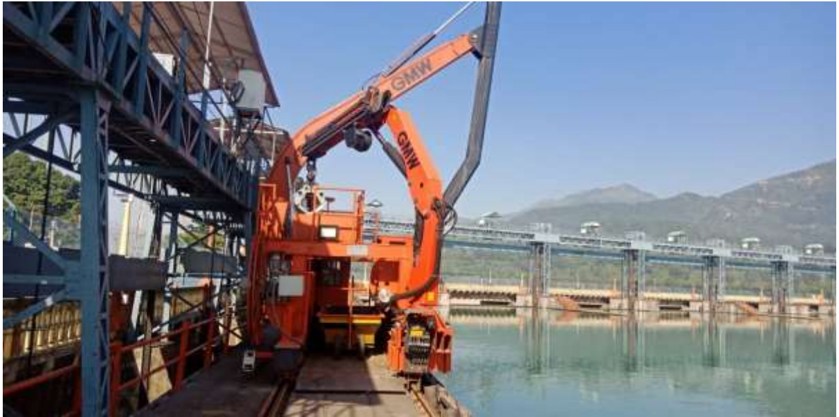
Trash rack cleaning machine after Installation
