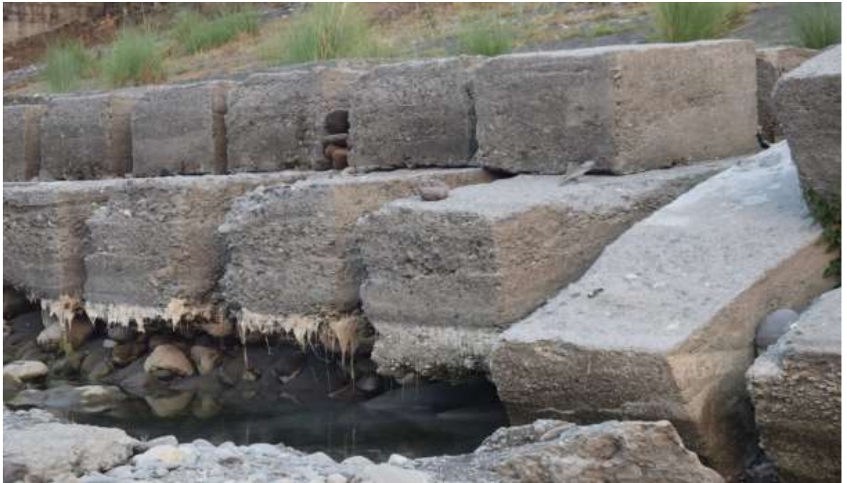
Status of protection works at downstream left bank before repair works
