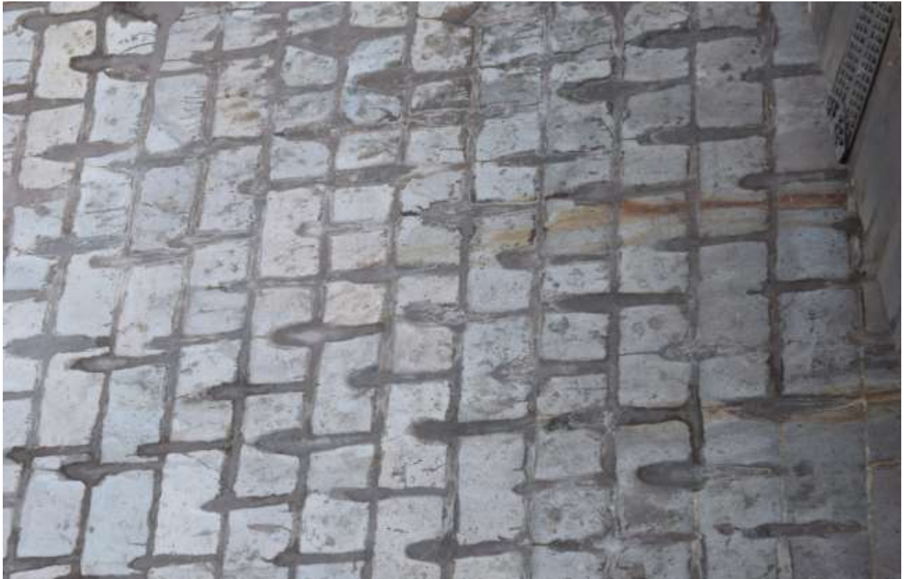
Status of downstream glacis after repair works
