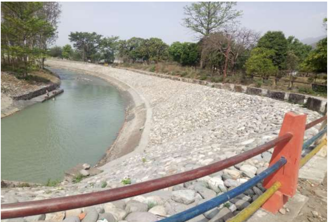
Status of right bank of silt ejector channel after repair works
