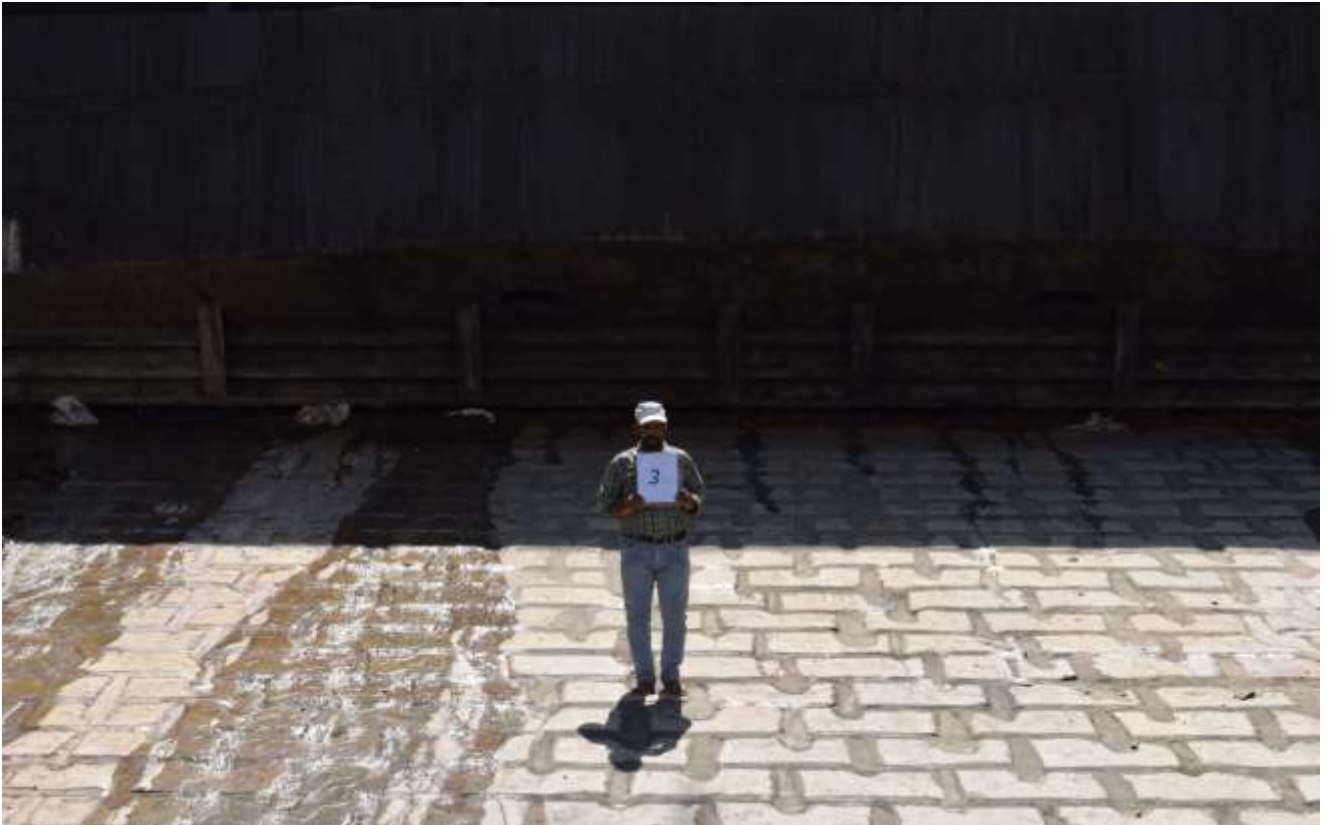
Status of downstream glacis after repair works
