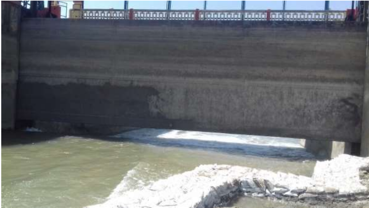
Barrage gates before epoxy painting
