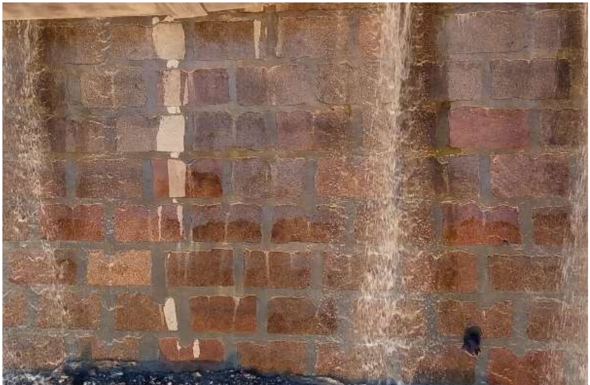
Status of upstream glacis after repair works
